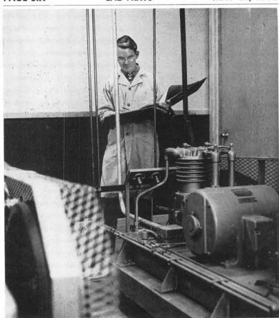
POWER FOR THE helium refrigerator is supplied by these two 15 hp compressors. Above, Gary Krieger (1413-2) is monitoring the gauges which show pressure at different stages of compression.
